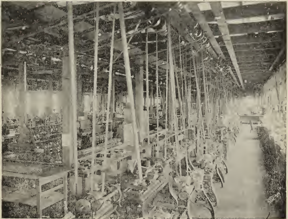
Main Machine Shop—350 feet long—General view—Edison Phonograph Works.
